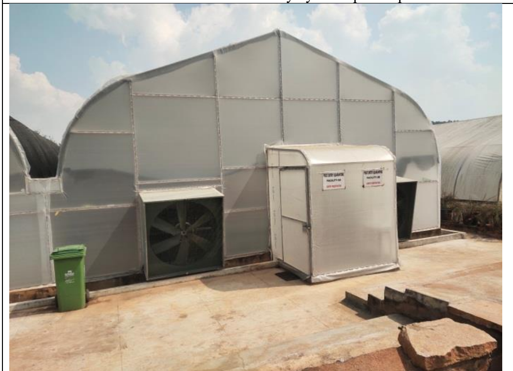
A post Entry-Quarantine (PEQ) Facility at Bangalore
